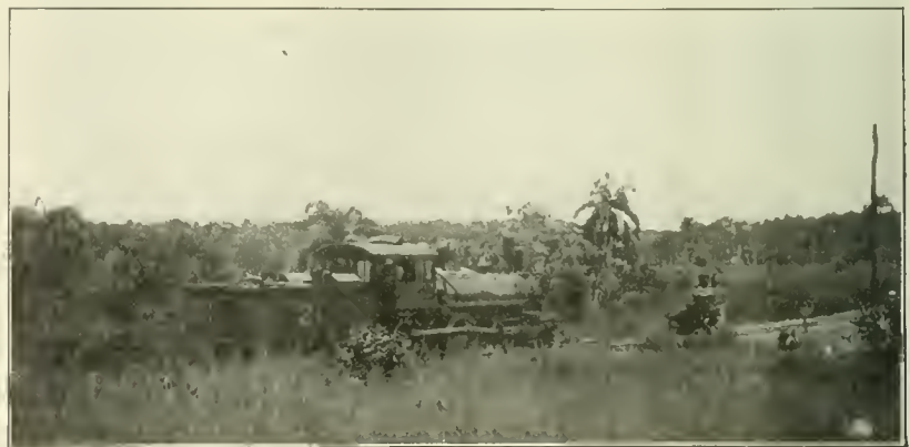
WORK TRAIN AND INSPECTION CAR.
